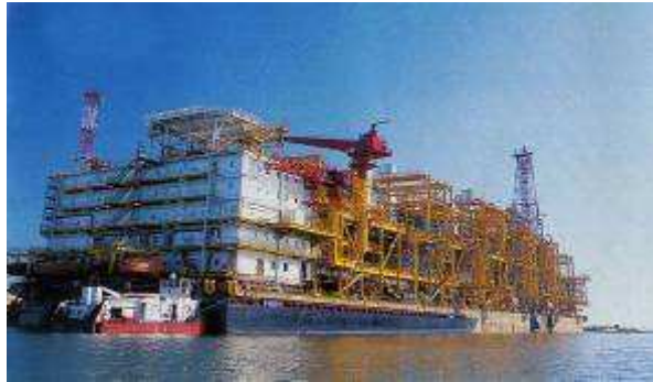
Elf Nkossa - Floating Production System (FPS) - oil & gas platform with LPG extraction - 30,000T topsides with concrete hull
